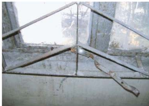
No maintenance of moving parts of window
